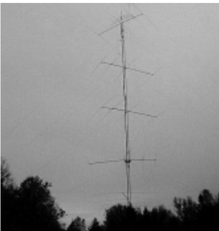
K1TTT 4/4/4/4 20 m stack on a 150' tower
