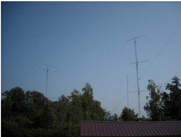
Left to right at W1AW/KL7: 15-meter stack, 160-meter vertical, 20-meter stack (Photo - Ward Silver NØAX)
