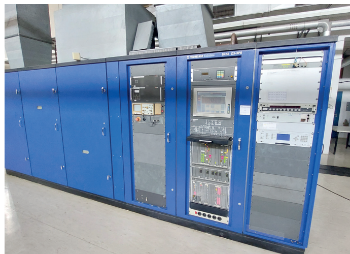
Thomcast 250-kW-SW-Transmitter
